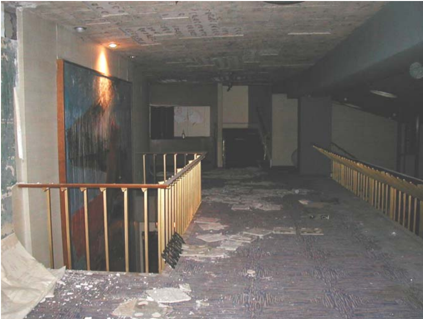
The mezzanine stairs to the upper balcony had also been filled in with gypsum block.
