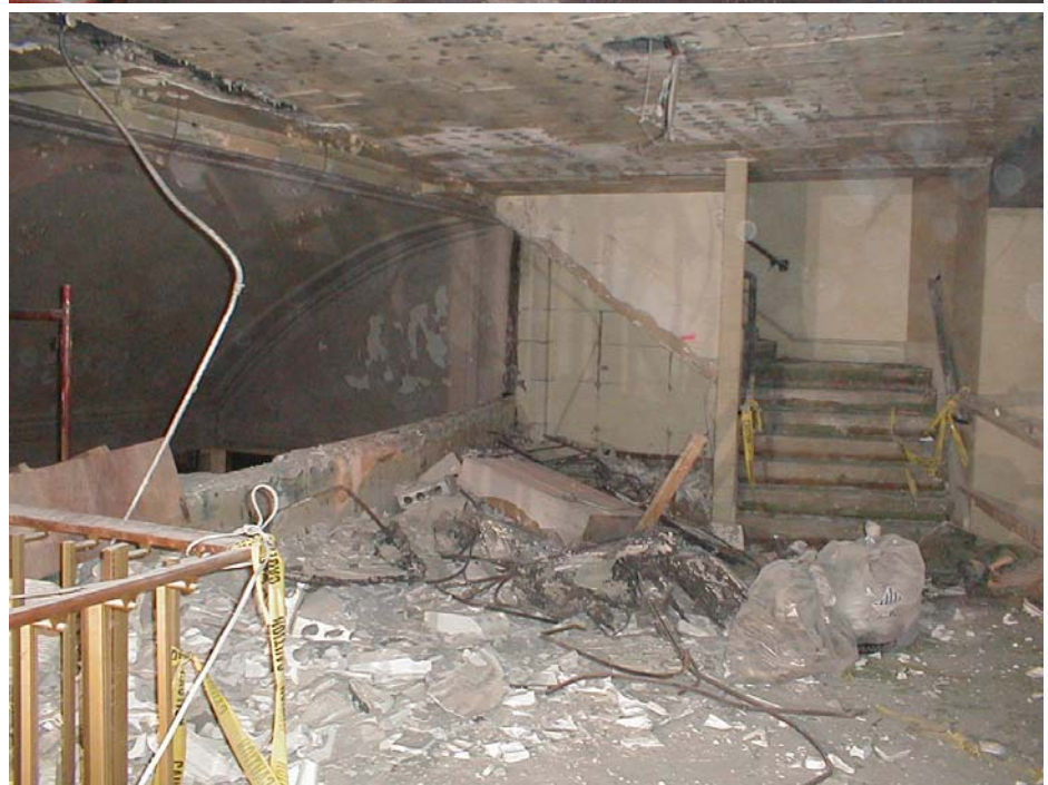
The mezzanine stairs to the upper balcony had also been filled in with gypsum block.
