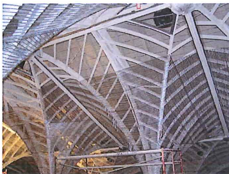
Ribbed lath was used to replace the wood lath because of its stiffness and ability to span between the supports.
