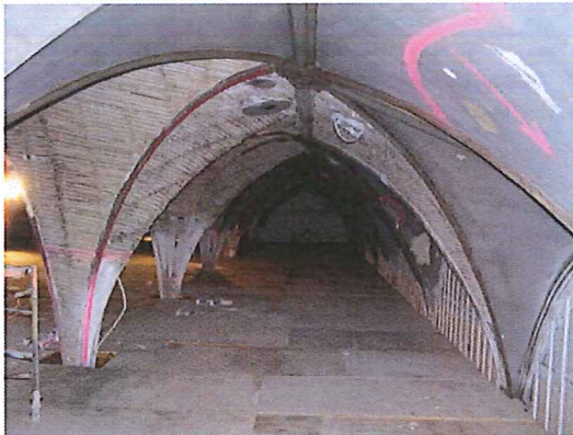
Removal of plaster revealed the wood laths that had been nailed in place 150 years before. Note the "dance floor" staging built high above the sanctuary to expedite the renovation.
