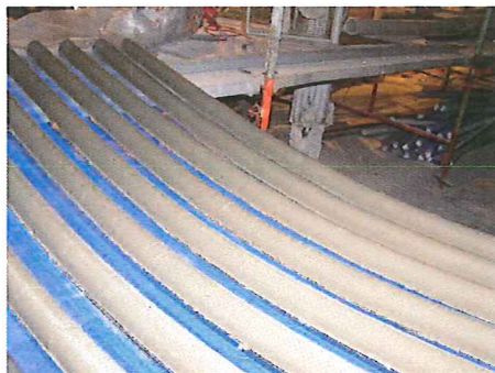
Expanded polystyrene was used to replicate the rope plaster moldings dividing the vaulted ceiling into panels.
