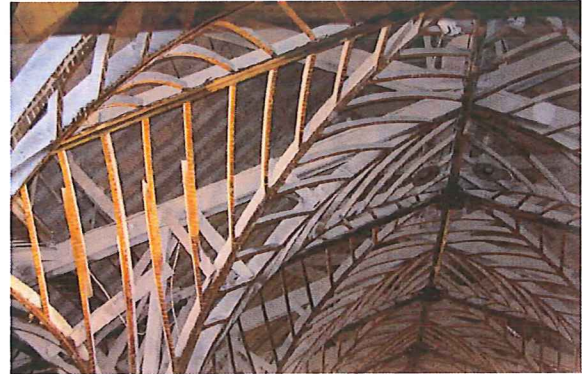
The wood framework skeleton that supported the complex ceiling.
