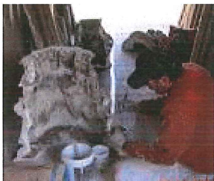
Making silicone molds of the original capitals with angel sentinels.
