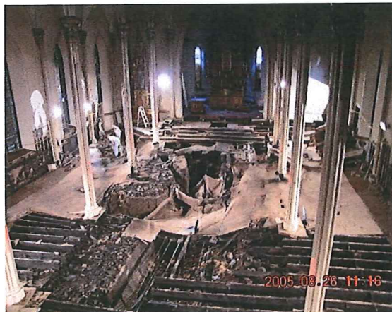
The fire smoldered and consumed most of the floor over a period of eleven hours.
